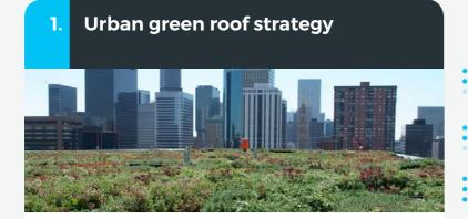
Green roofs within urban environments can reduce the runoff of water into the city's sewerage system, while at the same time, mitigate the urban heat island effect. Incentivisation programmes under a municipal green roof strategy can boost the implementation of green roofs through subsidies and other fiscal incentives.
