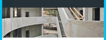
To overcome the prejudices of, and stimulate market demand for, recycled concrete in construction, the State of Berlin clearly specified the use of recycled concrete in the construction of a new University building. The tender reduced 880m² of virgin materials, as well as 66% of energy demand.<sup>18</sup>
